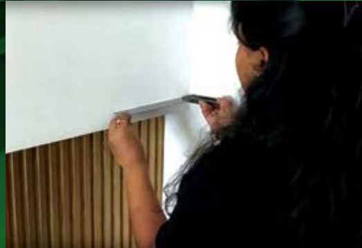
Nemmathi Team during their inspection▲
