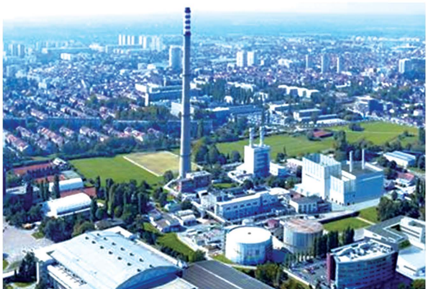
The Zagreb combined heat and power (CHP) site
