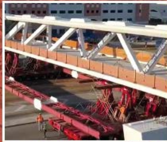
Fig. 3 Main span of the Pedestrian Bridge at FIU before, during, and after transportation
