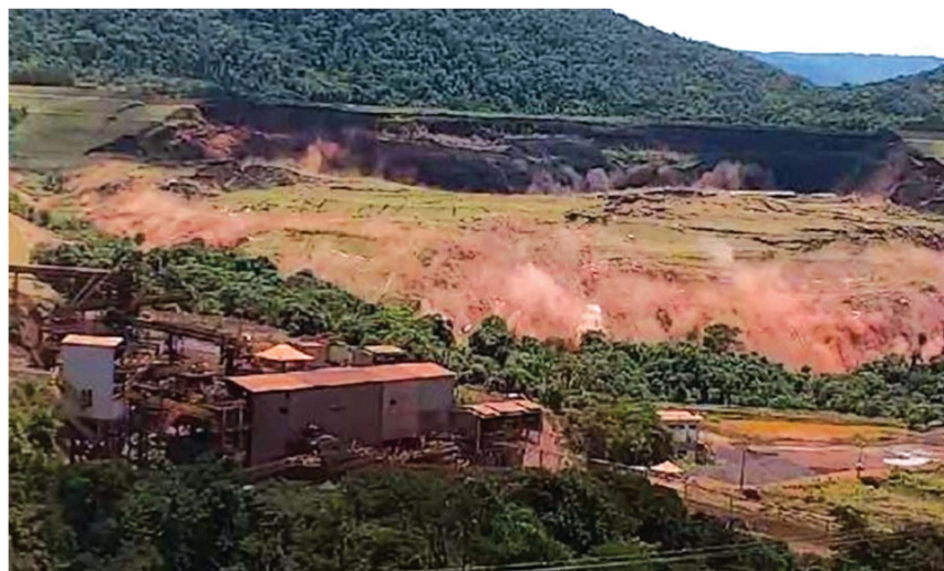
The collapse was caught on video, which helped the expert panel identify the causes.
